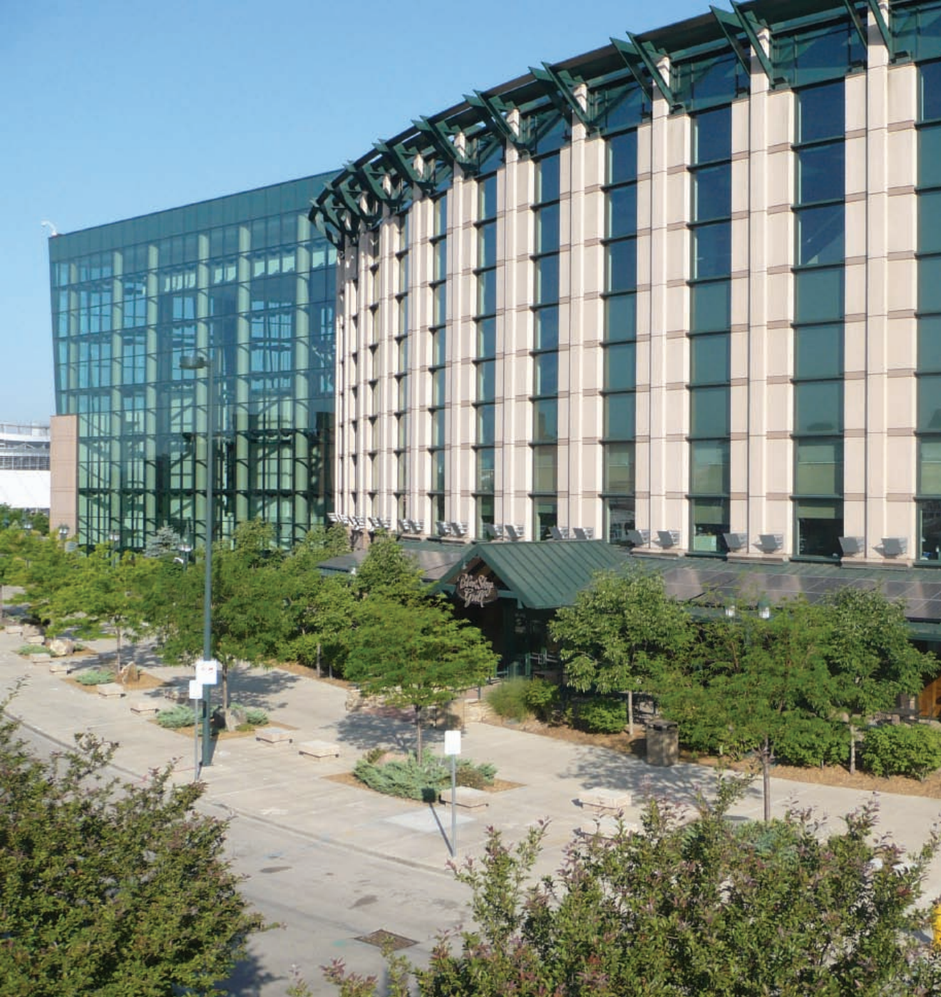
Denver-based SolSource Energy Solutions installed the 10-kilowatt photovoltaic system on the Pepsi Center, the first major U.S. sports arena to become carbon neutral.
