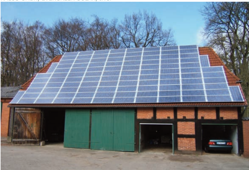
Germany has committed to installing renewable energy systems like this 12-kilowatt photovoltaic system on a farmer's barn near Buecken.
