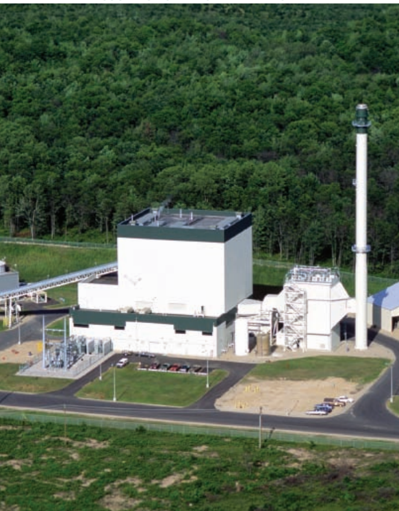
Left: The Grayling Generating Station burns biomass (waste wood), providing more than 36 megawatts of electricity to Grayling, Michigan, using a renewable resource. Right: A farmer fills up his tractor with Blue Sun FUSION™ B20 biodiesel.
