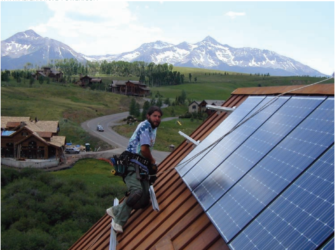
An employee of Ridgway-based Alternative Power Enterprises installs a photovoltaic system on a home in Mountain Village, Colorado, in 2007.
