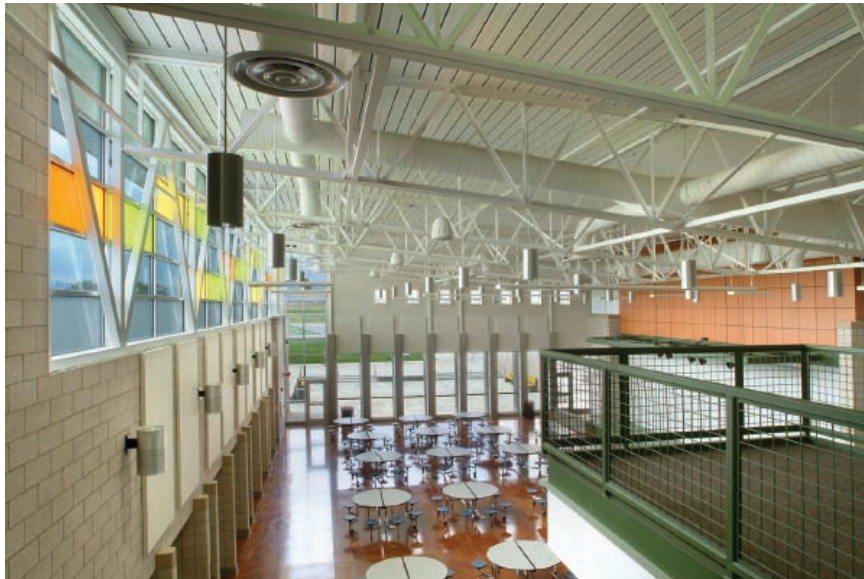
EMS Engineers provided mechanical engineering and commissioning services for the high performance, award-winning Kinard Junior High School in Fort Collins, Colorado.
