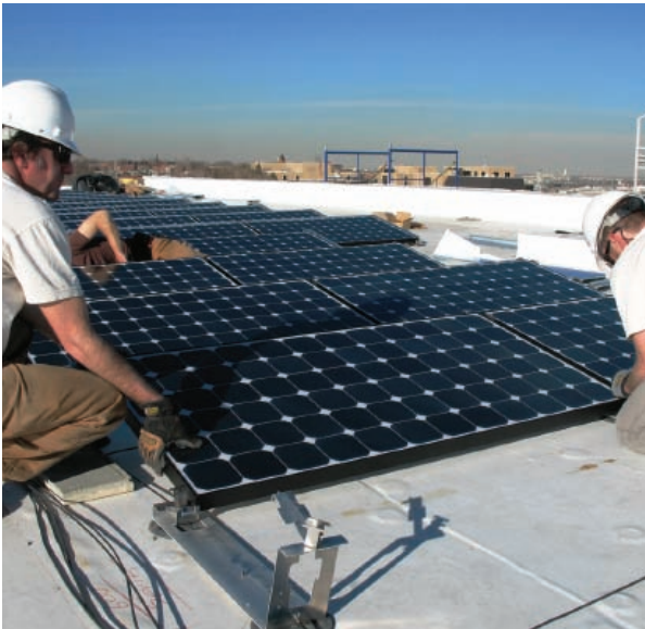
Left: Employees of Boulder-based Namaste Solar Electric install a photovoltaic system at the River Clay Condos in Denver; Right: A worker installs Johns Manville blown-in fiberglass insulation to improve the energy efficiency of a new home.
